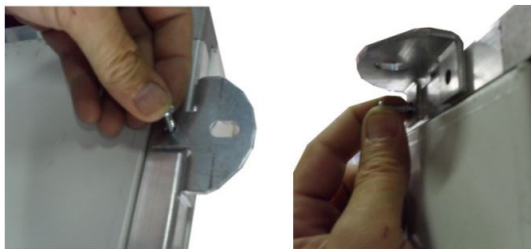
Fig. 1 - Fastening with the supplied brackets
